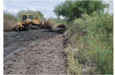
Dozer working on Sibley's Pond
